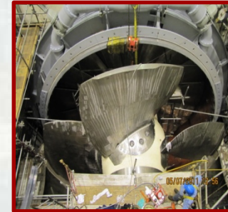
Webbers Falls Turbine
